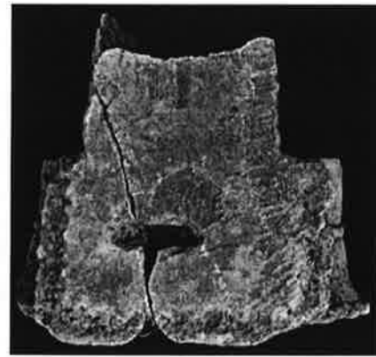
Fig. 17.11. Agora Gate. Unfinished moulding at joint.
