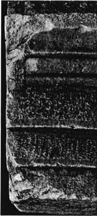
Fig. 17.12 (above). Sebasteion. Propylon, podium crown moulding, with unfinish at joint.
