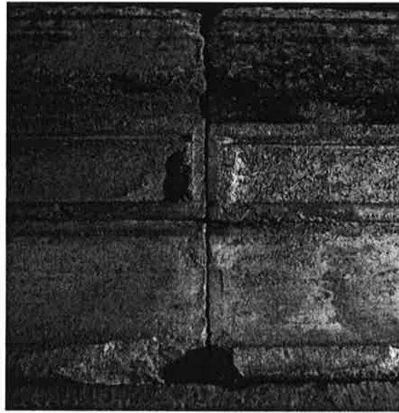
Fig. 17.12 (above). Sebasteion. Propylon, podium crown moulding, with unfinish at joint.
